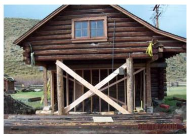
2) To rebuild the wall, new logs or repaired ones were stacked from from top down in a gravity defying act! The initial stabilization effort on the repaired south wall is visible in the photo at left.
