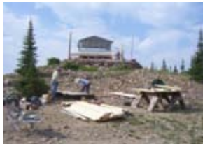
Basin Butte Lookout Work in Progress
